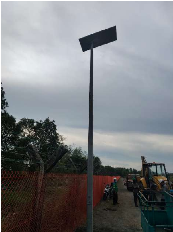
All in One TNB Station Kapar, Selangor
