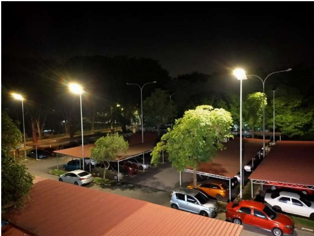
All in One Jkr Selangor Quarters
